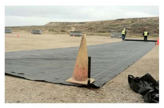
Geotextile is recommended for Supa-Trac HeliPad applications:
