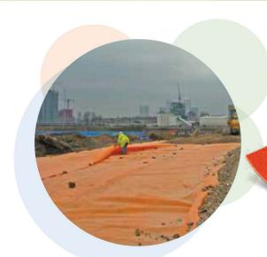
TERRAM Hi Vis is a non-woven orange geotextile used for separating contaminated/uncontaminated soils.
